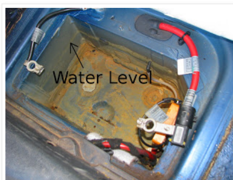
Battery Compartment half filled with water
